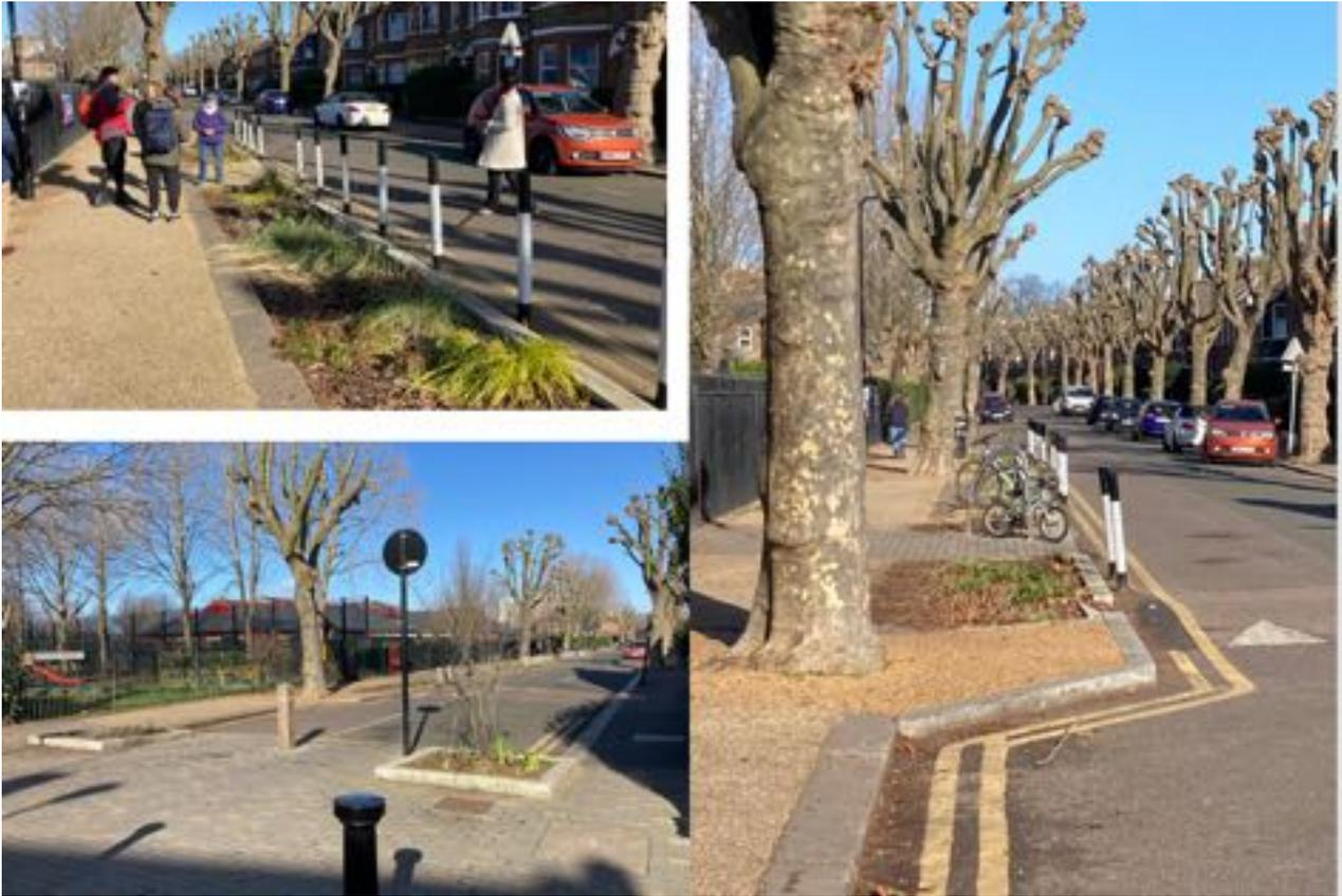
Buildout of pavement (protected by wands); road filtered to eliminate rat-run traffic; planting / Sustainable Urban Drainage System (SUDS).
