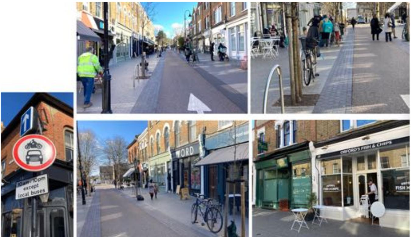
The road now has a 'bus and cycle gate' allowing only bus and pedal cycle entry between 10AM and 10PM; pavements widened; car parking removed; cycle parking added; carriageway flush with footway. This has become a very successful shopping and eating street with higher retail occupancy than previously.
